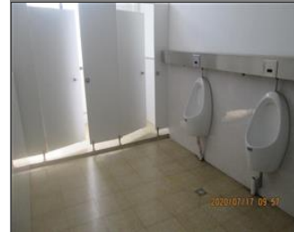
Photo of the sanitary facilities toilets.JPG
