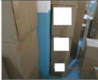
Photo of non-conformity NC The packing materials were stored close to the columns.JPG
